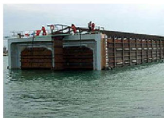
Fig. 8: Marmaray Crossing, Turkey
