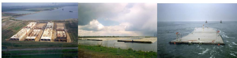
Fig. 2: Tunnel elements in casting basin, in flooded casting basin and during offshore transport (Piet Heintunnel, The Netherlands)
